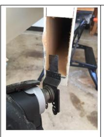
Marked the cut-line with the "decapitated" base moulding and used a multitool with ¾" wide blade to remove the defective MDF strip. Slid a thin putty knife between the outside panel and the multitool cutting blade to prevent accidental damage to the panel.
